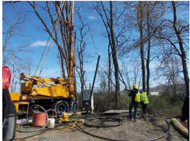
Workers remove the steel well casing from a former schoolhouse site and restored the area.
