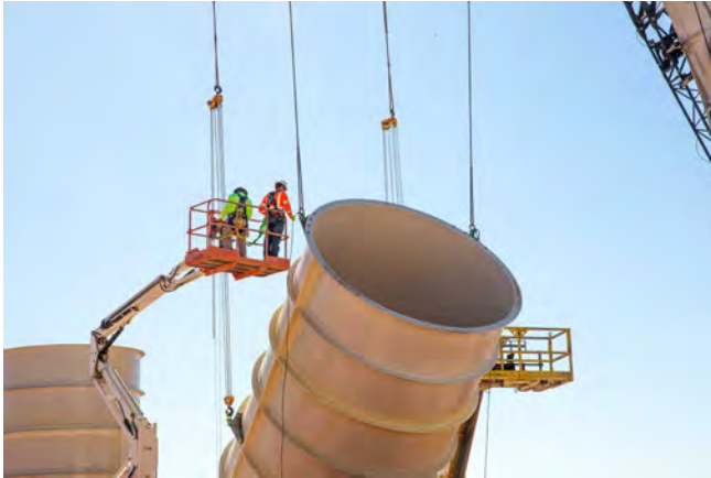
Workers attach guiding tag lines to ductwork before lowering it into a channel adjacent to the utility shaft at WIPP.
