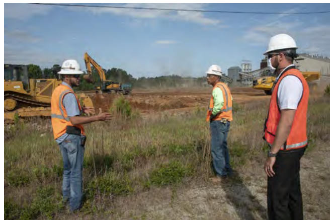
SRS completed the D Area Coal Yard cleanup project to excavate and blend soil with fine-grade limestone to lower pH levels.
