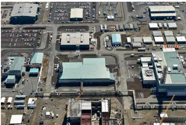
Commissioning of the DFLAW Program facilities took a giant leap forward in November, when the WTP completed startup testing of all systems needed to transform low-activity tank waste into a safe form for disposal.
