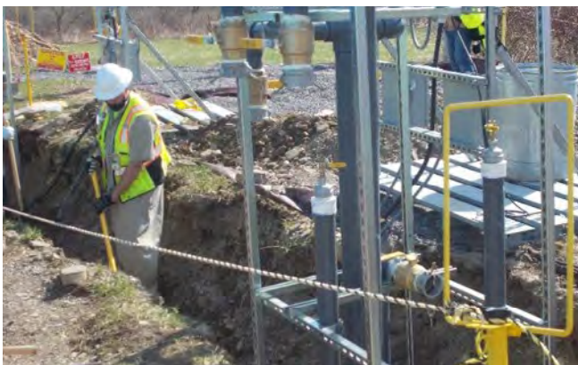
Crews install a robust water management system in preparation for MPPB demolition.
