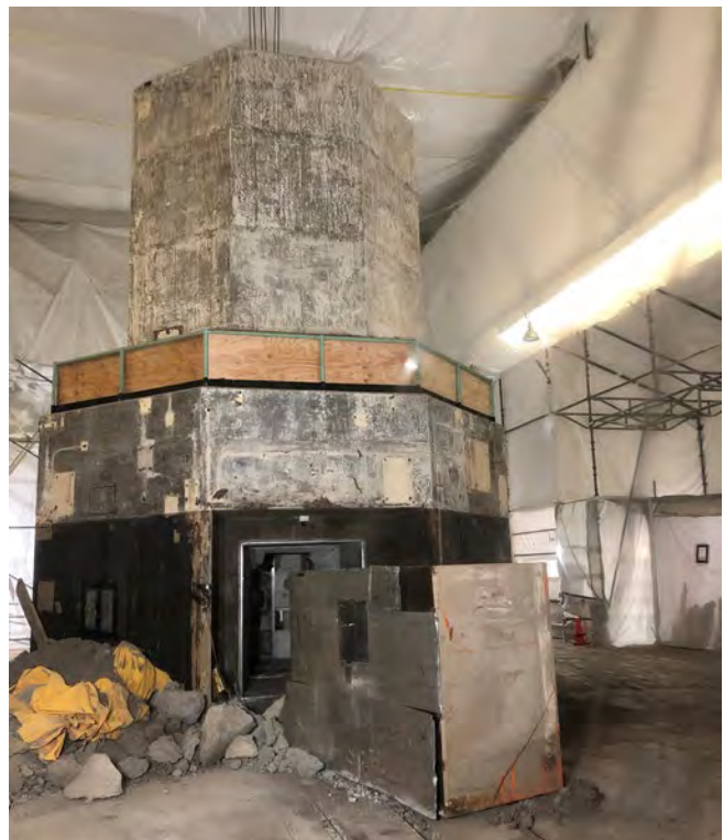
Building 280 reactor's west thermal column door during demolition.
