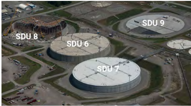
SRS continues to meet mission needs by constructing mega-sized SDUs to permanently dispose of decontaminated saltstone.
