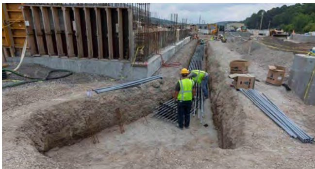
View of construction progressing at the Mercury Treatment Facility. When operational in 2025, it will be able to treat up to 3,000 gallons per minute.
