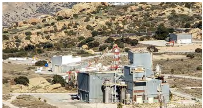
ETEC before final building demolition.
