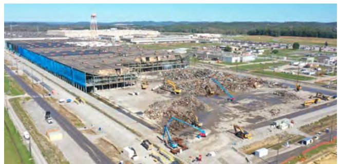
Demolition of the X-326 process building began in May.
