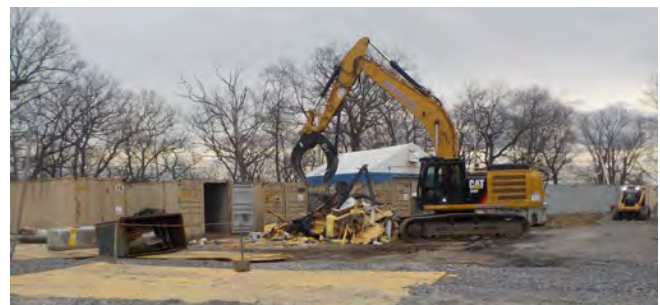
Removal of F-Yard excess materials.
