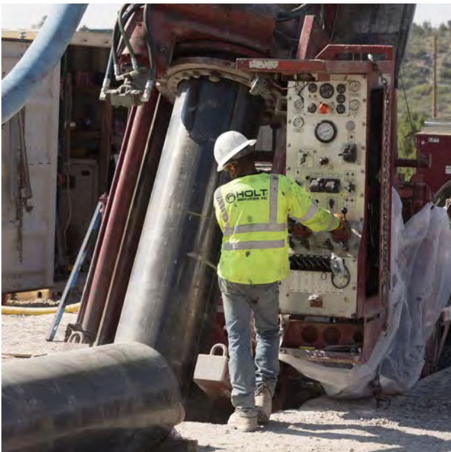
A drilling contractor advances casing during construction of Well R-71.
