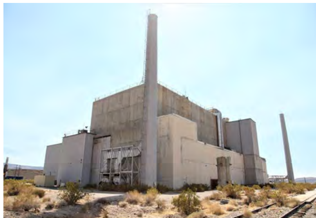
Characterization is underway in preparation for demolition and closure of the EMAD facility.
