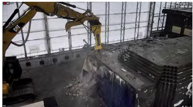
Crews remove the former Radiological Development Lab's West Cell Bank at ORNL. Crews built a protective cover over the structure to ensure a safe teardown of the high-risk contaminated structure.
