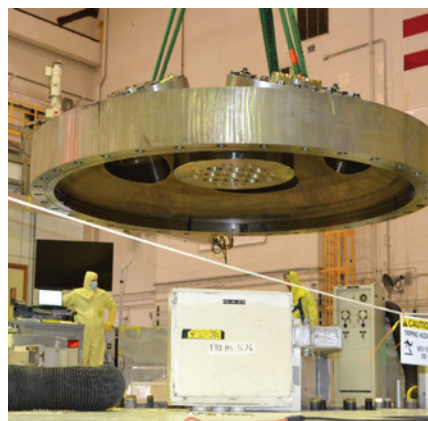
Reactor top head installation during CIC-VI
